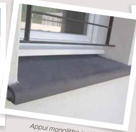
*Appui monolithe isolé*
